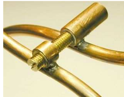
A home made capacitor with Delrin insulation was getting hot.
